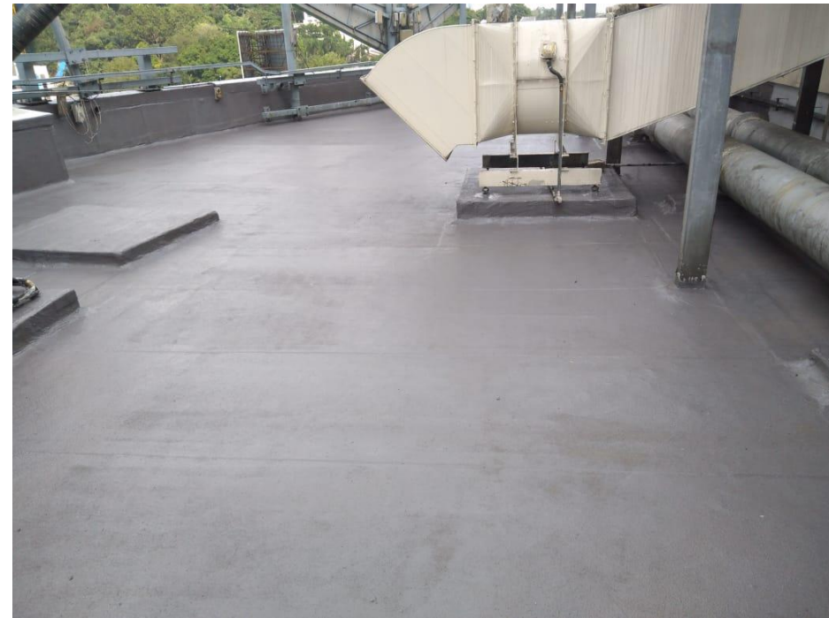
North Rooftop Waterproofing
