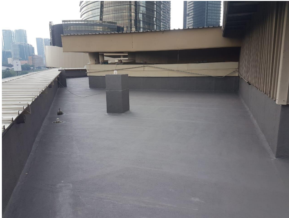
South Rooftop Waterproofing
